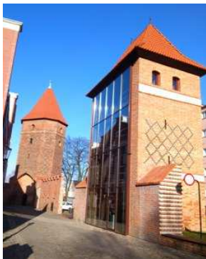
Pic. Ramparts with towers
